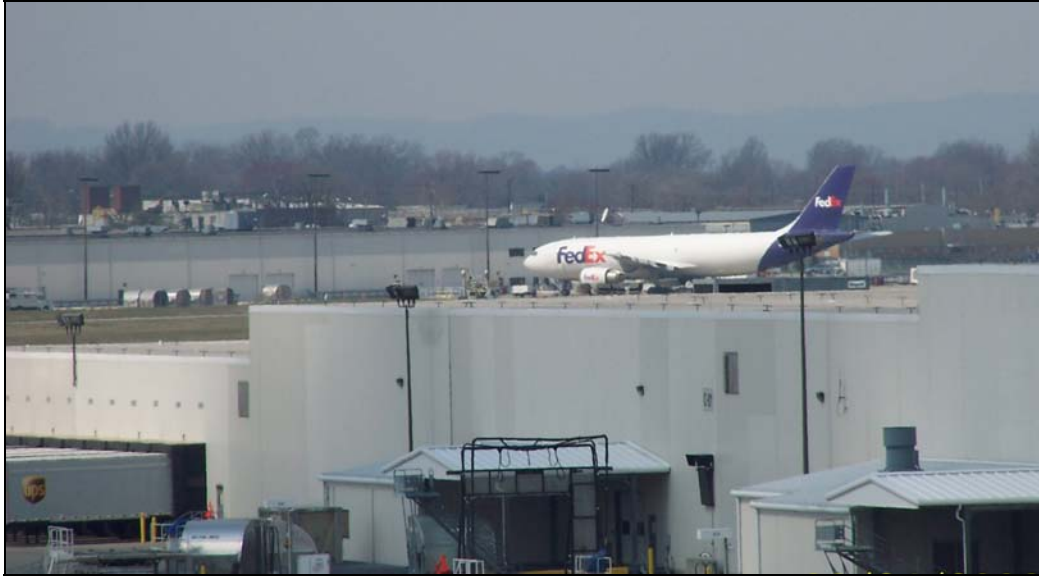
Figure 12 Contiguous UPS and FedEx Facilities
