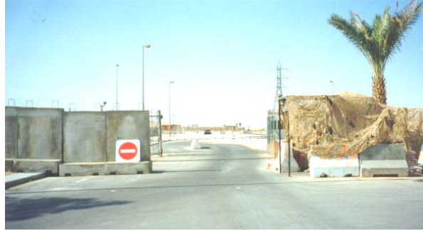
Figure 3.12. Bitburg Barriers Employed for Counter-mobility
