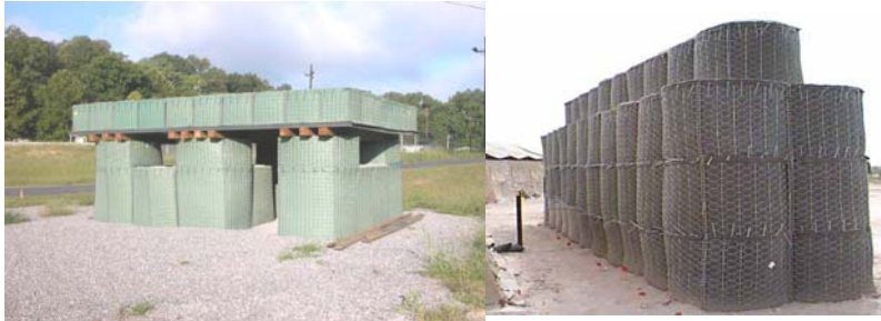
Figure 3.15. Concertainer Styled Barriers Used as Blast Walls and Fighting Positions (Concertainer Construction Techniques per ERDC Guidance)
