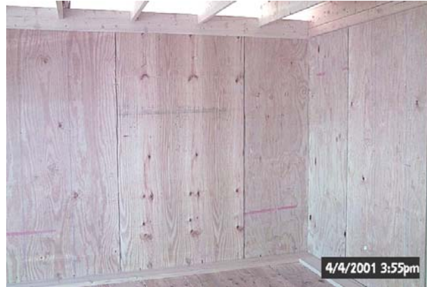
Figure A4.42. Overall View of Retrofitted SEA Hut
