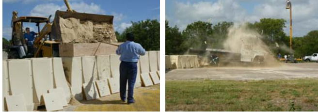
Figure A4.20. Sand-filled Plastic Barriers
