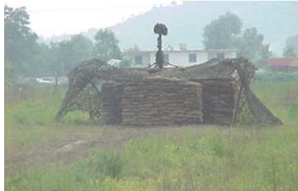
Figure 3.13. Sandbags Used for Fragment Protection
