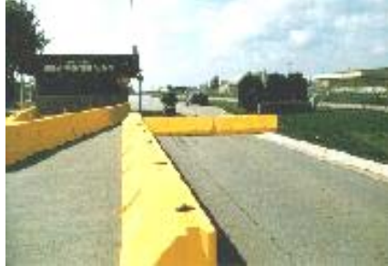
Figure 3.14. Water Filled Barriers Used for Counter-mobility
