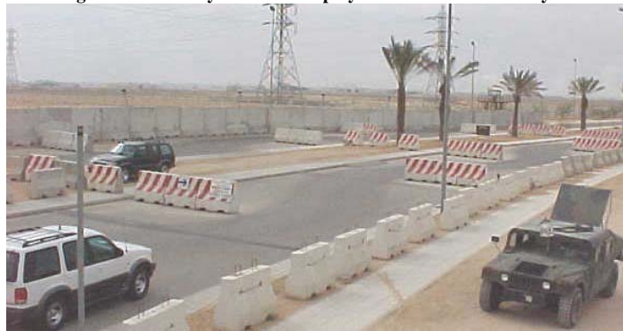
Figure 3.11. Jersey Barriers Employed for Counter-mobility
