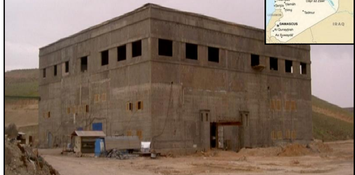
Al Kibar Reactor
