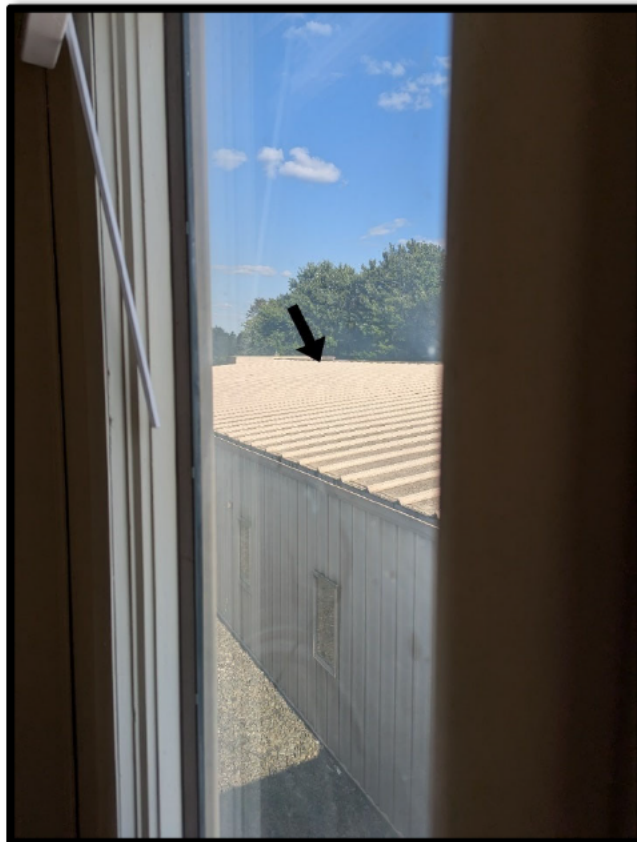
View looking left from AGR building breakroom 116
