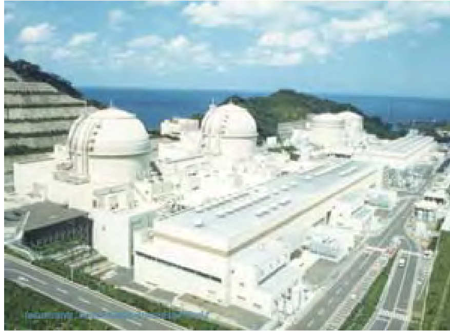
Figure 49 Ohi Nuclear Power Station, Ohi-cho, Fukui, Japan
