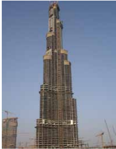
Tower under Construction
