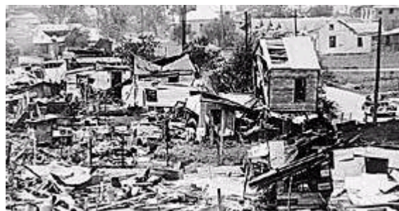
(U) Damage to Texas City was extensive, as indicated by these damaged and destroyed houses
