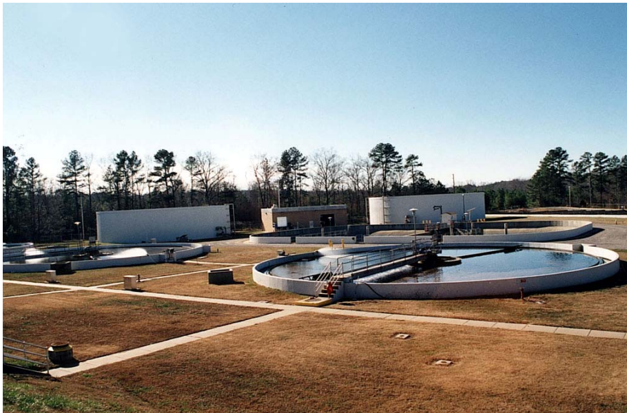
Figure 8 Wastewater Clarifier
