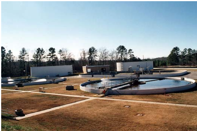
Figure 7 Wastewater Clarifier
