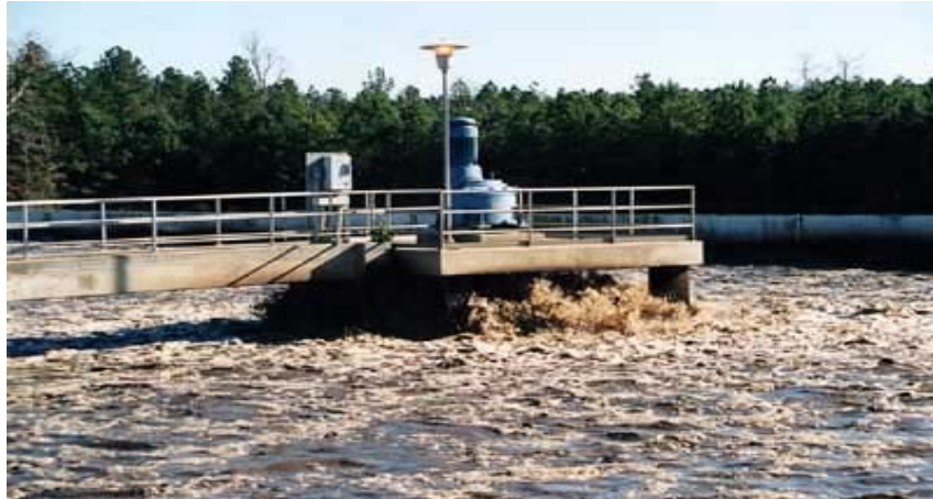
Figure 6 Wastewater Aeration Basin
