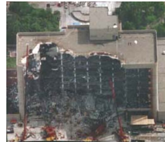
Damage to the Federal Office Building, Oklahoma City, from a Truck Bomb
