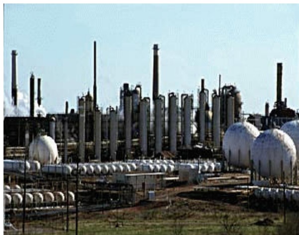
Figure 1 Oil Refinery Showing Distillation Columns
