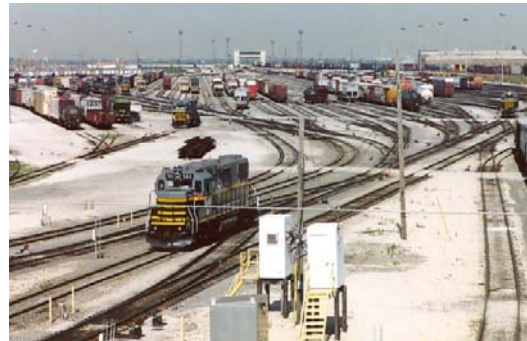
Figure 3 Rail Yard Illumination by Day
