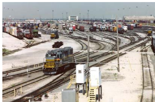
Figure 2 Rail Yard Illumination by Day
