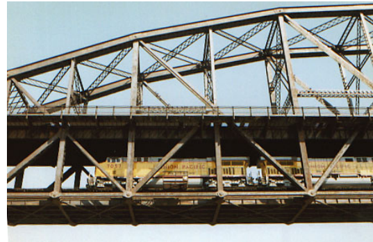
Figure 2 Bridge with Overhead Highway
