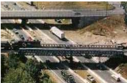
Figure 1 Railroad Bridge over Highway
