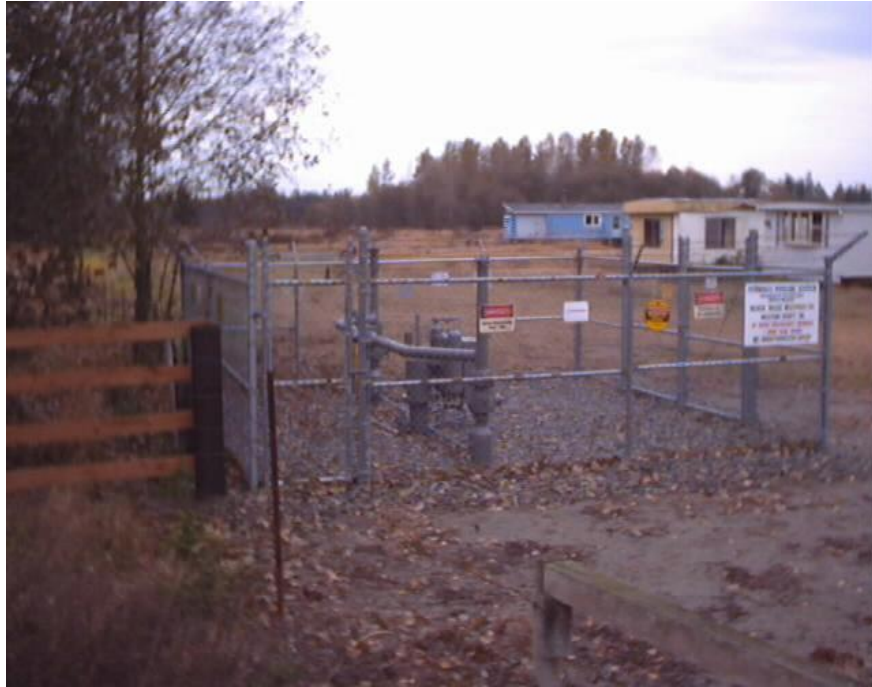
Figure 7 Typical Block Valve Station and Enclosure
