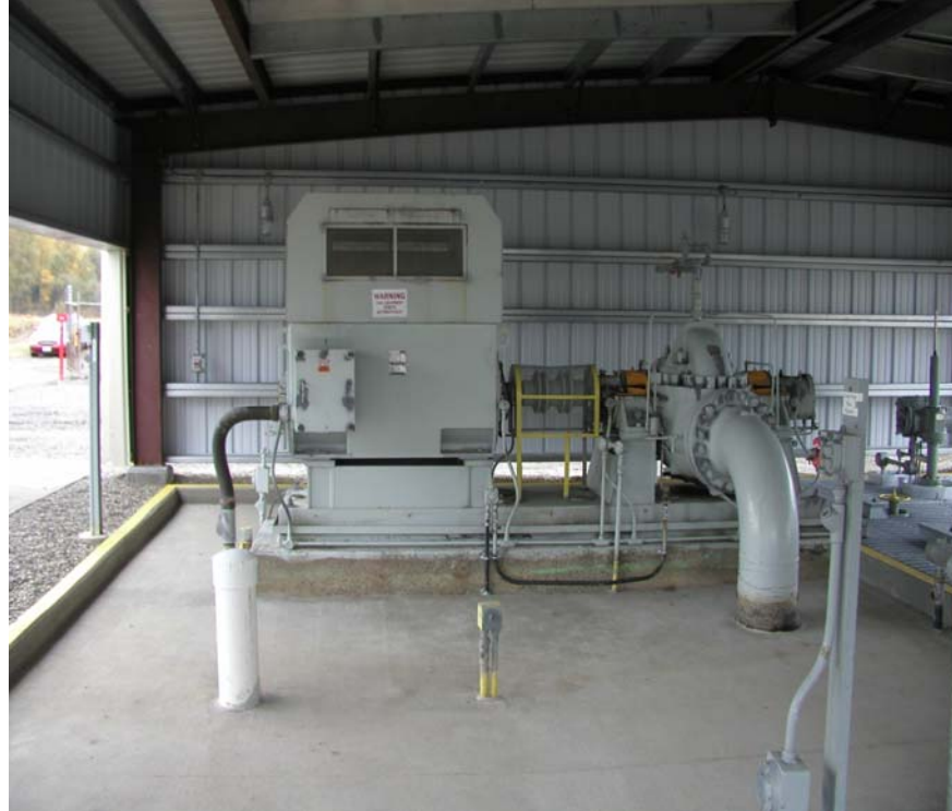
Figure 5 Inside View of a Pipeline Pump Station
