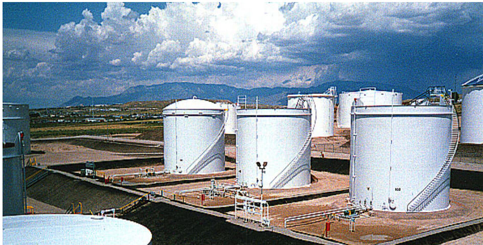
Figure 6 Typical Petroleum Storage Tank Farm
