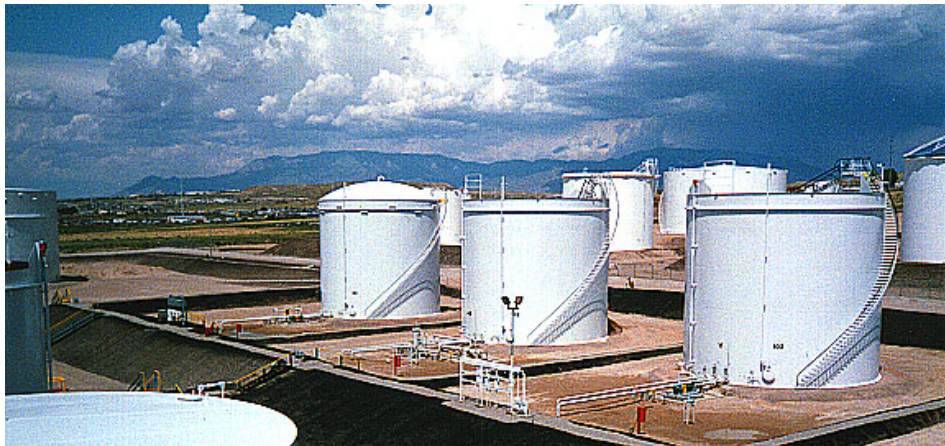
Figure 5 Typical Petroleum Storage Tank Farm
