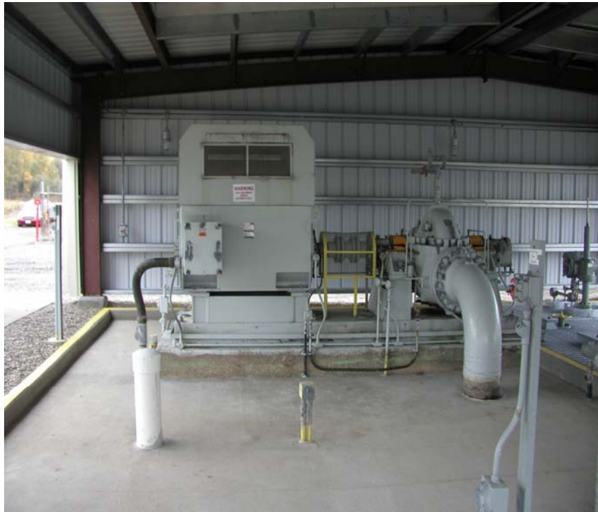
Figure 4 Inside View of a Pipeline Pump Station
