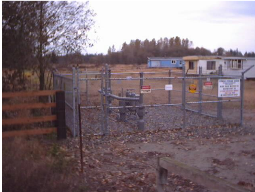
Figure 6 Typical Block Valve Station and Enclosure
