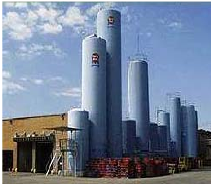
Figure 5 Storage Silos for Raw Milk
