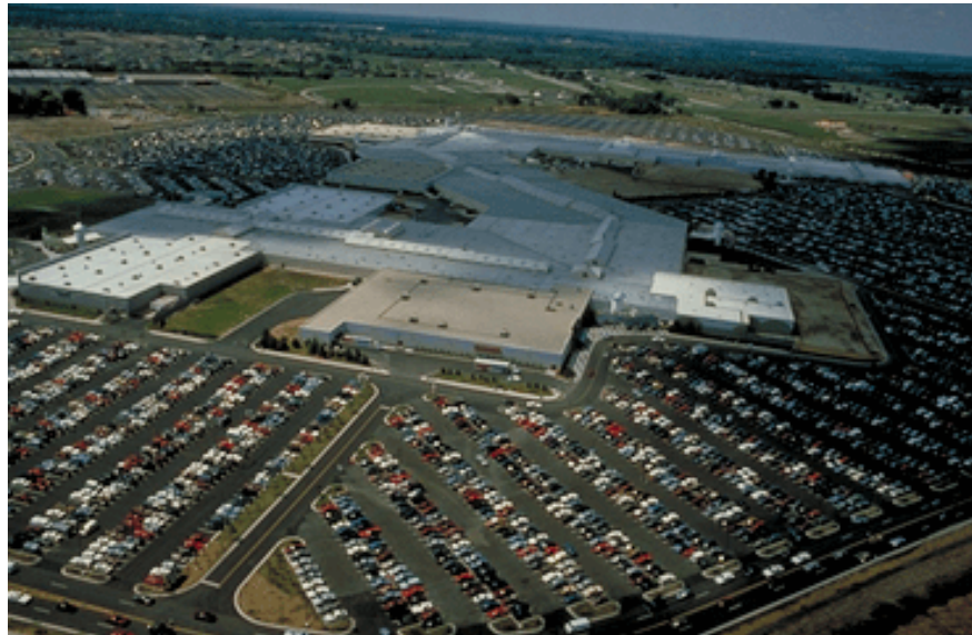
Figure 3 Typical One-story Mall and Its Surrounding Parking Lots
