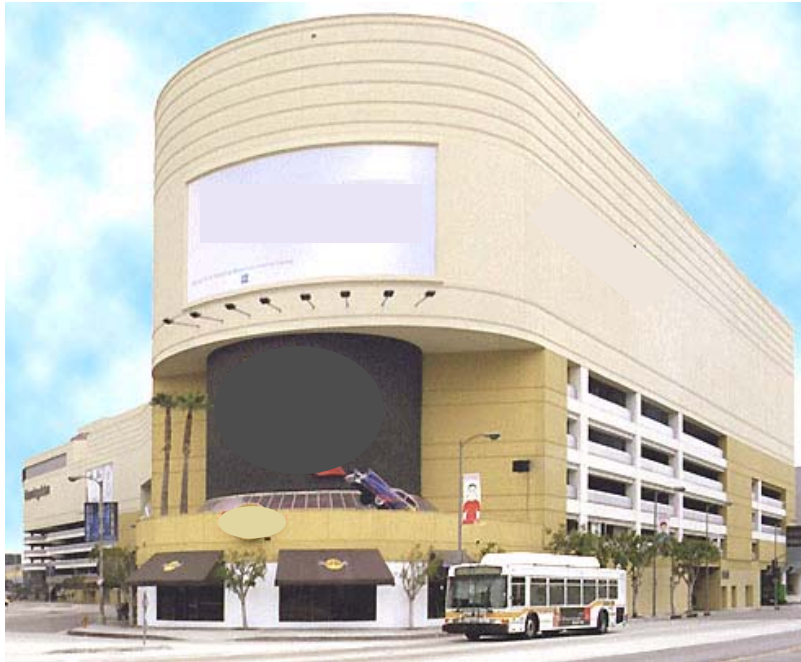
Figure 7 Typical Mall Indoor Parking Garage
