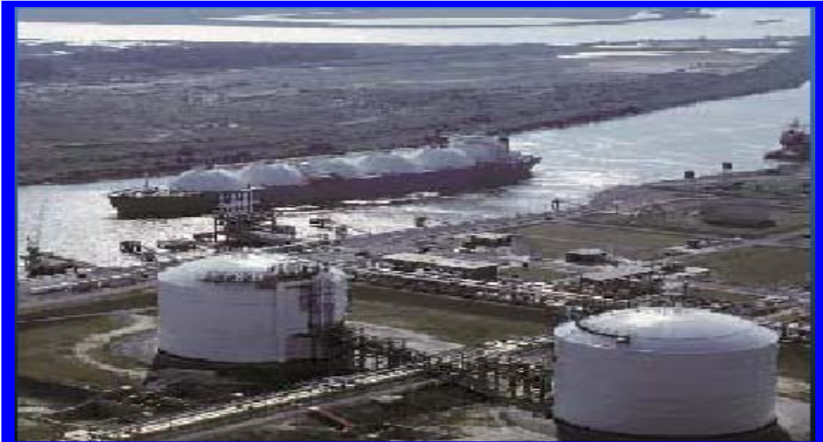
Figure 1 Lake Charles, Louisiana, LNG Import Terminal (Source: Quillen 2002)
