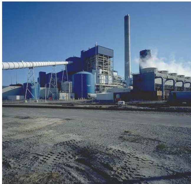
Figure 2 Modern Coal-Fired Steam Power Plant
