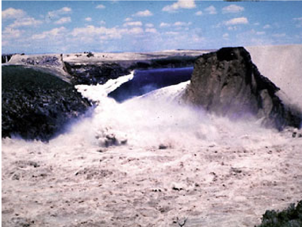
Figure 4 Failure of Teton Dam in 1976
