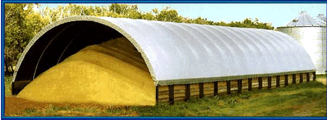
Figure 3 Local On-Farm Grain Storage
