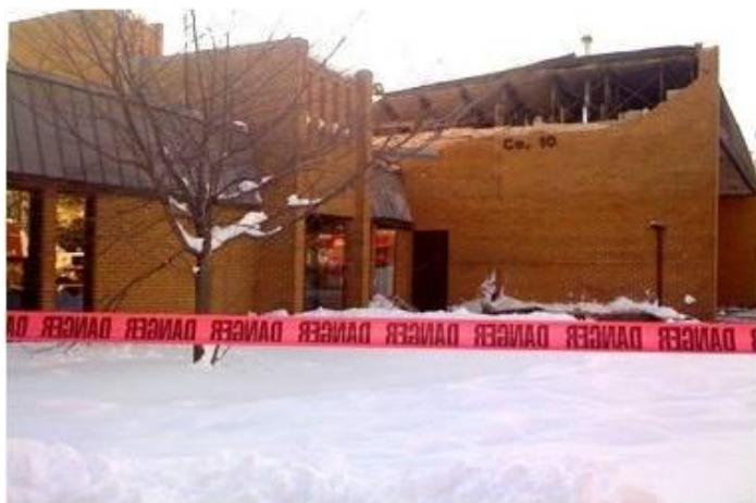
Roof collapse in Virginia at the Fairfax County Fire Department following heavy snowfall in February 2010.
