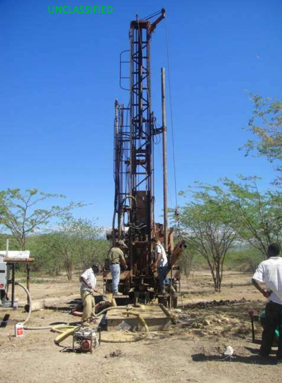
Drilling 2 nd Well IOT create additional water point
