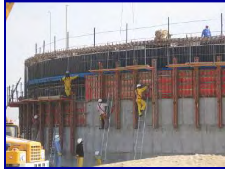
Raising Bulk Storage Tanks Exterior Lifts
