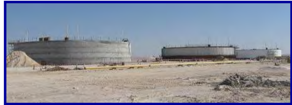
Bulk Storage (3-50K barrels, 2.1M gal ea)
