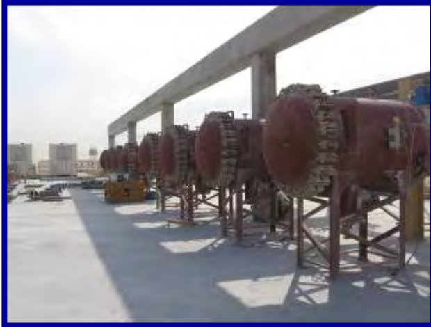
Bulk Storage Filter/Pump Installation
