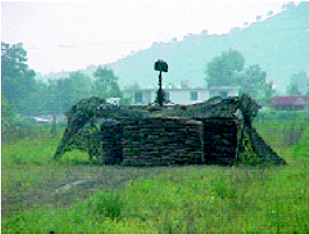
Figure E-4. Sandbags Used for Fragment Protection
