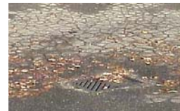
ALLIGATOR CRACKING
