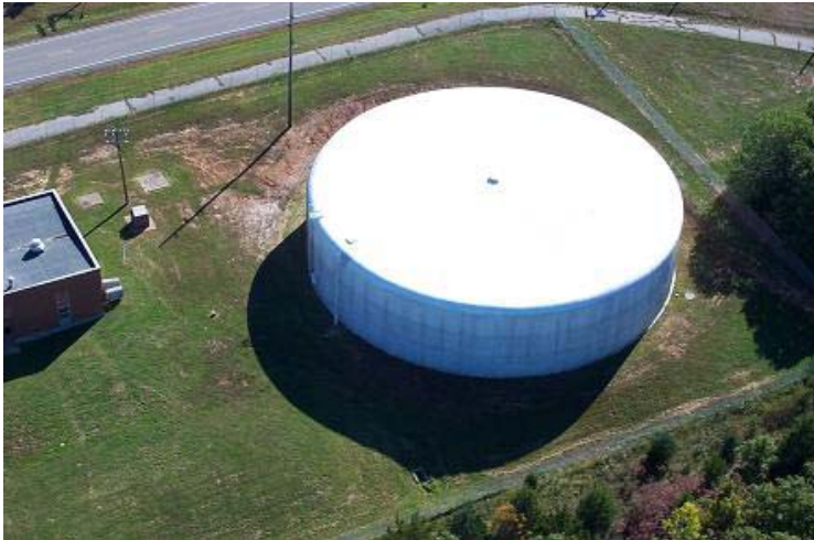
Ground level tank
