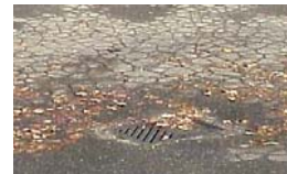
ALLIGATOR CRACKING
