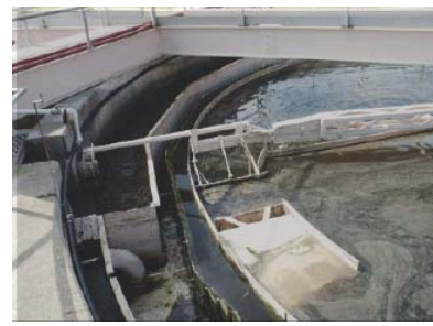
Secondary sedimentation tank and clarifiers
