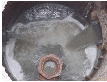
Junction box and cleanout
