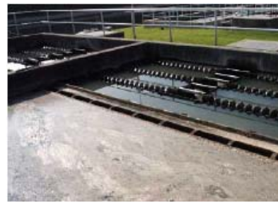
Primary sedimentation tank and clarifiers
