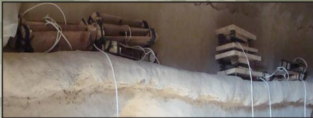
Cache - Various PPs Under Construction
