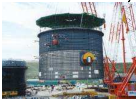
RCCV Lower Liner Module:630ton
