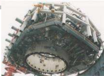
Upper Drywell Module:650ton
