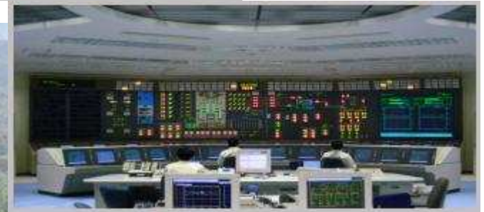
Main Control Room
