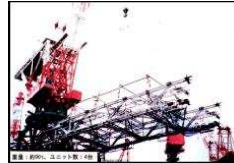
Roof Truss Module
