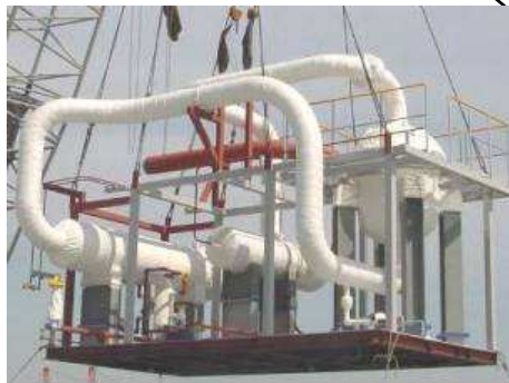
Off Gas Module
