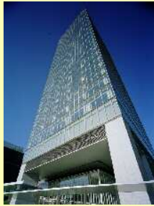
Nuclear Systems Div. Tokyo Headquarter Office
