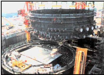
Reinforced concrete containment vessel (RCCV)
