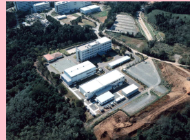
Power & Industrial Systems R&D Laboratory
