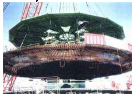
Base Mat Module:460ton
