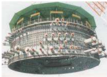
RCCV Upper Liner Module:170ton
