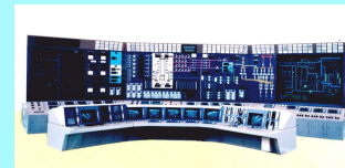
Main Control System
